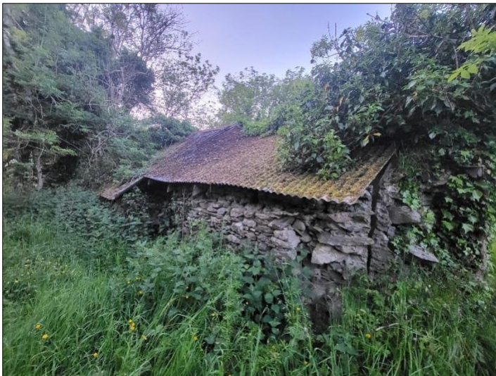
Figure 5. Rear view of the structure.
