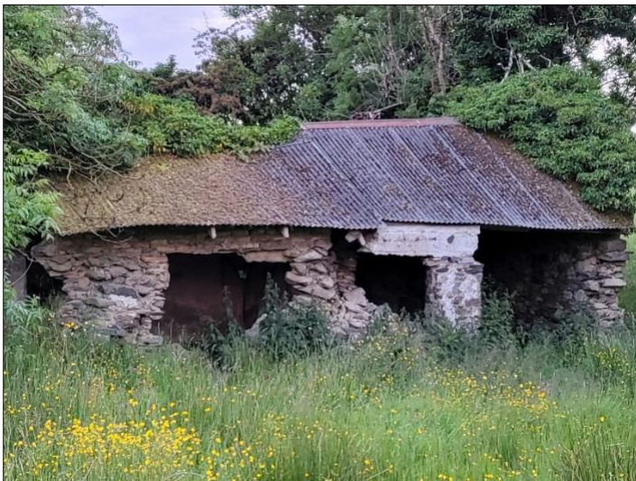
Figure 6. View of the front of the structure.
