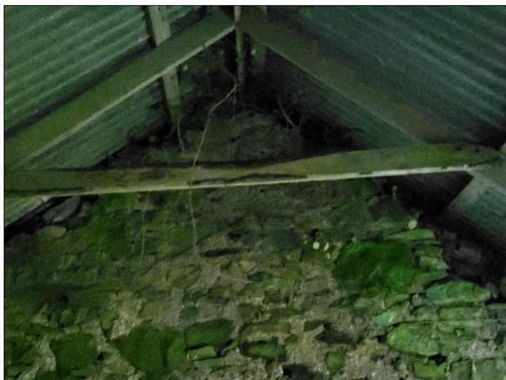
Figure 7. Internal roof timbers
