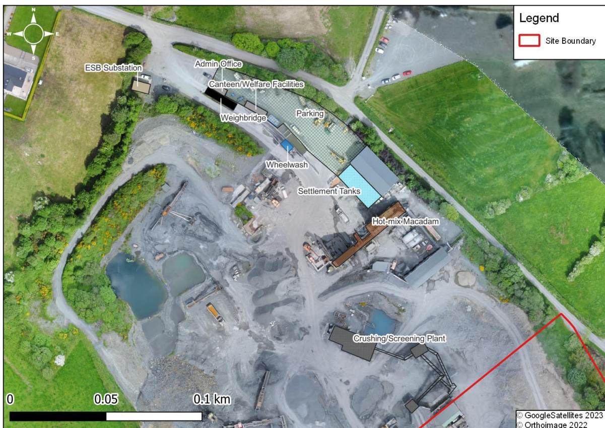
Figure 3-1: Scotshouse Quarry Infrastructure
